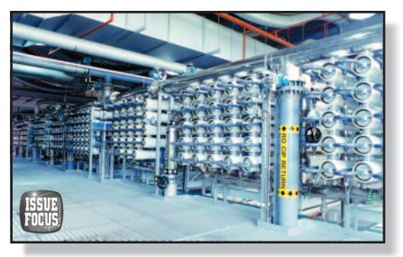
**RO reduction.** A new reverse osmosis water treatment system has been developed by O'Brien & Gere that the company says reduces the volume of discharge waste down to nearly zero percent. The units shown here are similar to those installed at an automotive facility in Saltillo, Mexico.
